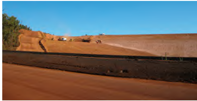
Tailings Storage Facilities
