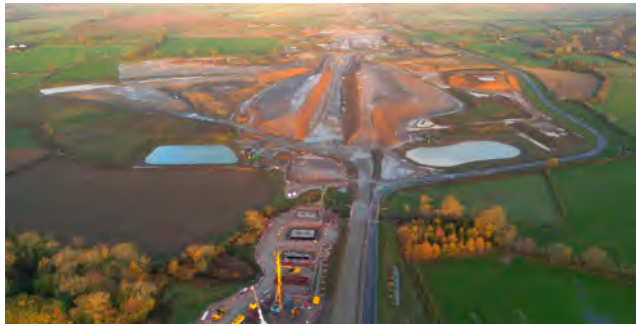
Road/ Rail Embankments
